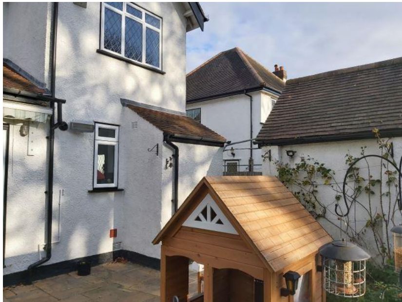
Photo 4. View towards rear of No. 35 wood Ride.
