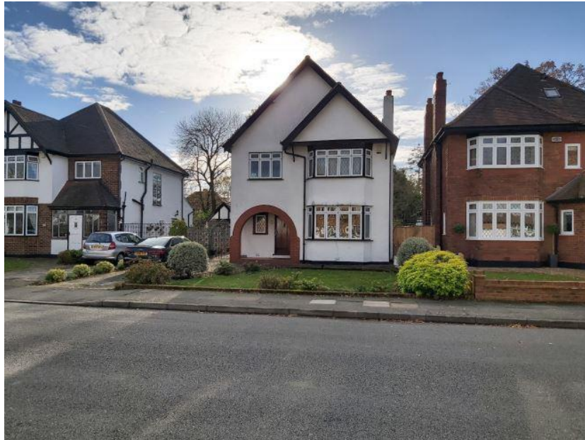
Photo 1. No. 37 Wood Ride (centre).
