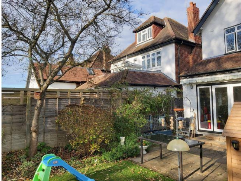
Photo 3. View towards rear of No. 39 Wood Ride.
